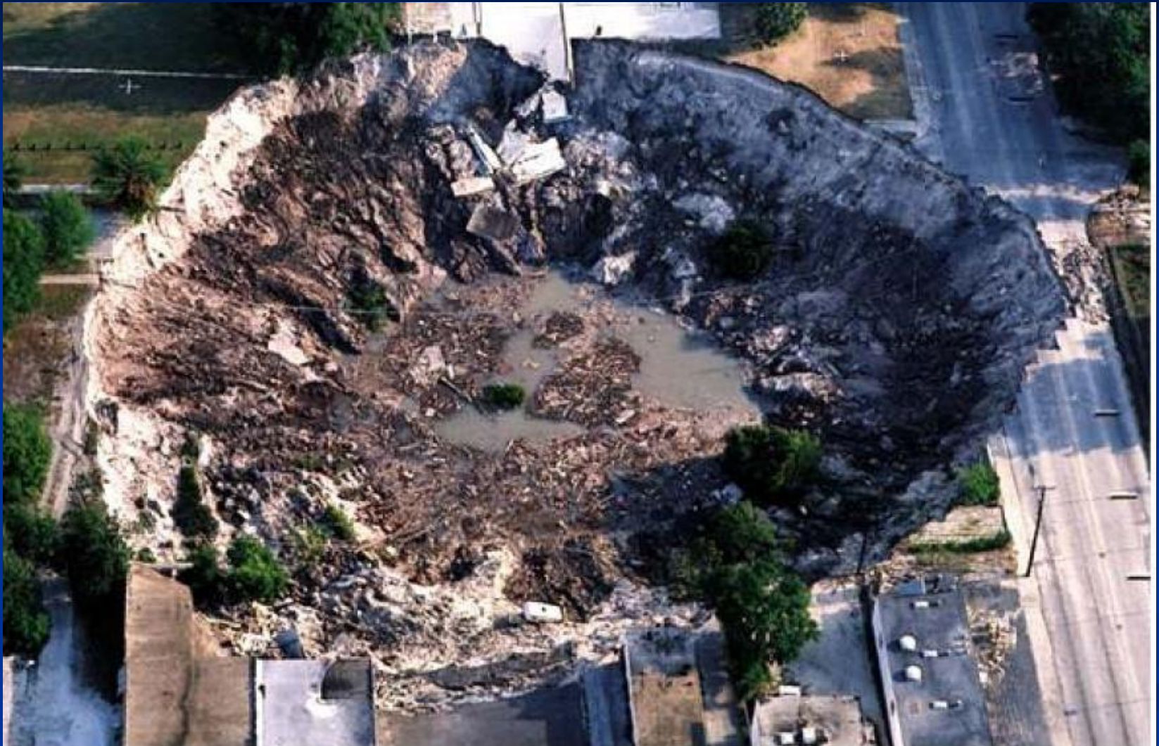
Winter Park sinkhole , Florida(1981)
